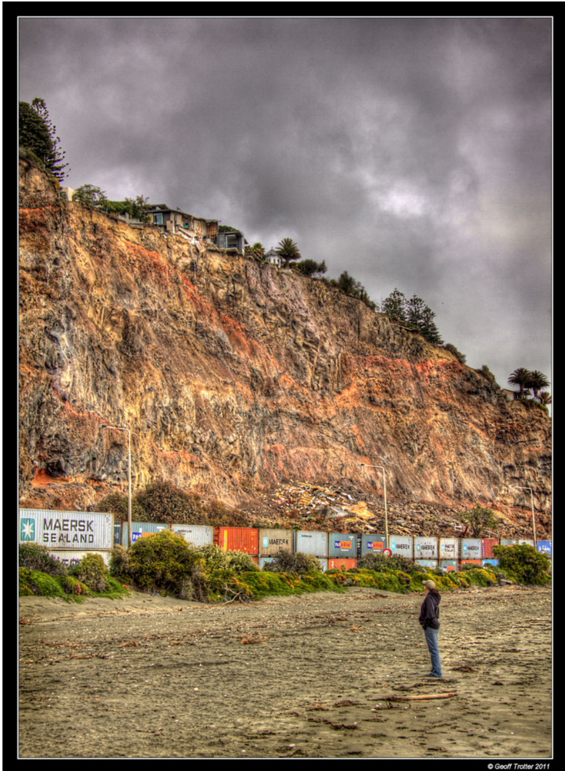
▲ Container train capturing ongoing rock falls, June 2011 — ©2011 Geoff Trotter
